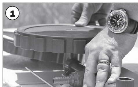
DO NOT USE TEFLON TAPE! Screw diffuser discs onto riser pipes, do not cross thread. DO NOT OVER TIGHTEN DISK.
