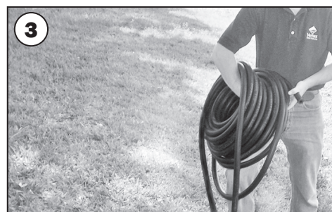
Uncoil supply tubing along the shore, making sure tubing is not twisted or tangled. Leave 4' tubing on shore and secure one end of the tubing so that it doesn't follow you into the water.
